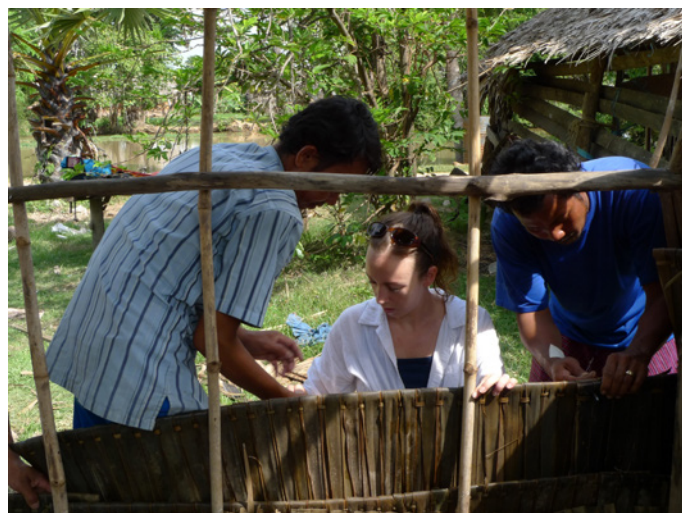
Building houses remains a common voluntourism activity, with wide variations in approach depending on the organisation. Here, volunteers in Cambodia rebuild a family home alongside local builders, with materials largely funded by the volunteers.
