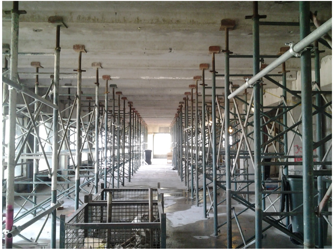
Structural propping during demolition of the Clarendon Tower
