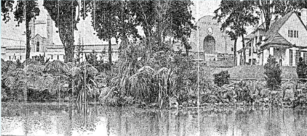
Figure 2. “The Exhibition Buildings from Across the Miniature Lakes,” New Zealand Herald , December 1, 1913. Note that the shape and position of the Concert Hall behind the Tea Kiosk could well have acted as a formal precedent for the Winter Gardens, see Figure 3.
