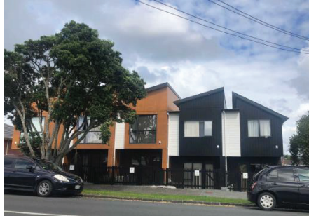
2 – street elevation facing East.
