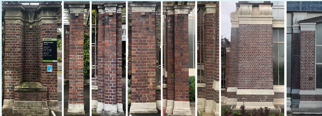
Figure 9. The many variations of the brick pier module in the Winter Gardens. Photos: Cameron Moore.
