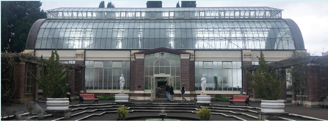
Figure 12. Glasshouse façade. Photo: Cameron Moore.
