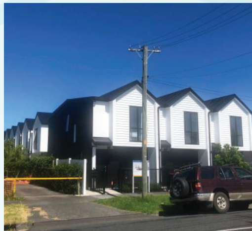
Figure 6. 26 Moa Road, Point Chevalier: nine 65m 2 two-storey terraced houses without on-site parking or service provision, developed at a density of 149du/ha. Photo: David Turner.
