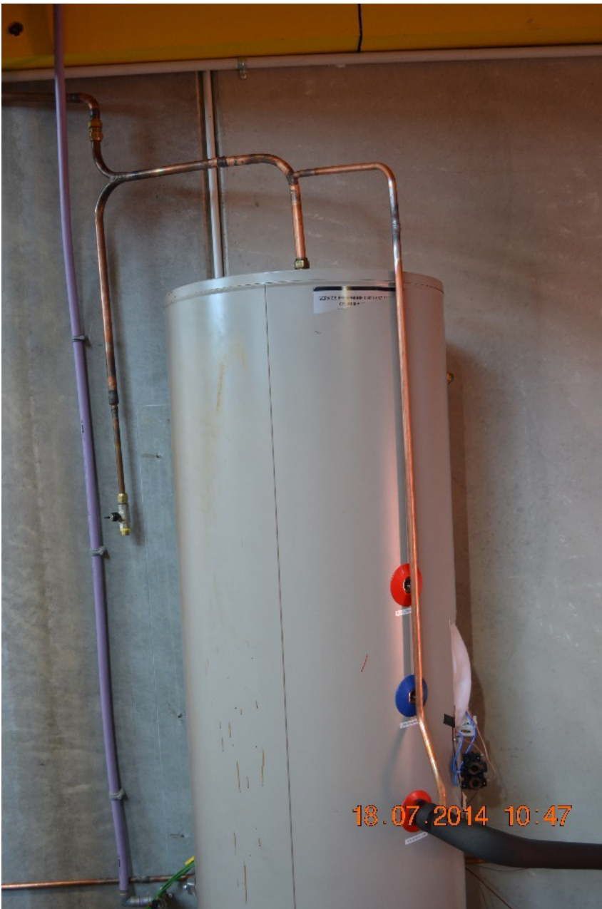
Figure 26. Stainless-steel indirect HWC, two coils.
