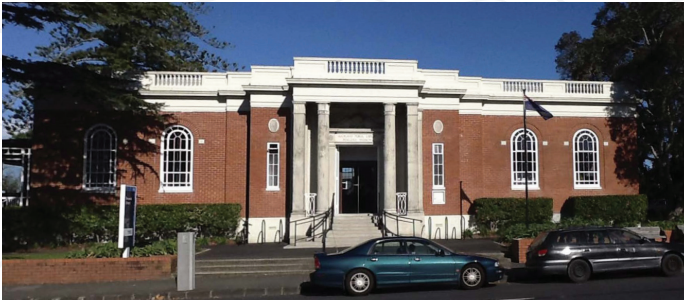
Figure 5. Remuera Public Library, architect William Gummer, 1926. Photograph by the author
