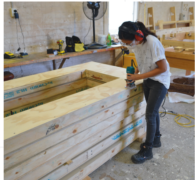
Figure 9. EDFAB 4.0 prefabricated panels being assembled and lined up ready for install onsite. Photographs: Yusef Patel
