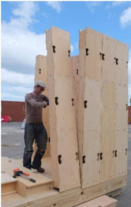
Figure 1. Above: The EDFAB 1.0 construction system. Below: The process of fitting the modules into position and locking them into place with the 'butterfly'.
