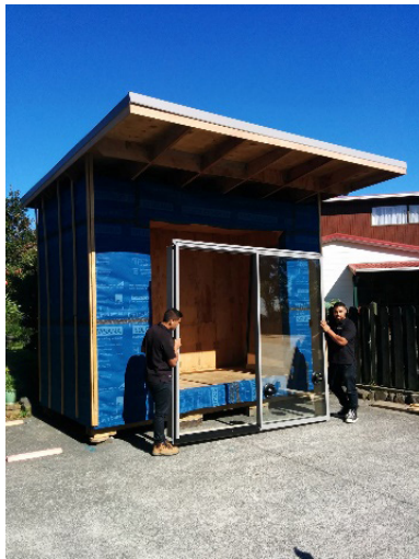
Figure 3. Smartfit window being installed, and the EDFAB 1.0 prototype completed on September 23, 2015, at a private residence in Manukau.
