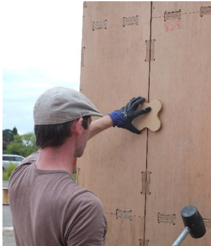
Figure 1. Above: The EDFAB 1.0 construction system. Below: The process of fitting the modules into position and locking them into place with the 'butterfly'.
