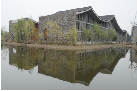
Fig. 5: Teaching Building No. 14, Xiangshan Campus Phase II, Hangzhou (2007) (Photo: Hing-wah Chau)
