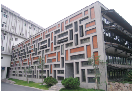
Fig. 2: Fig. 2 Teaching Building no. 21 in Phase II, Xiangshan Campus (2007). Photograph by Hing-wah Chau.
