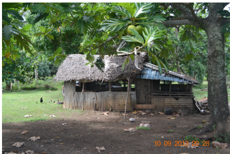
Fig. 10. Elevation of Kaho's Tongan kitchen now clad in corrugated metal, author September 2013.
